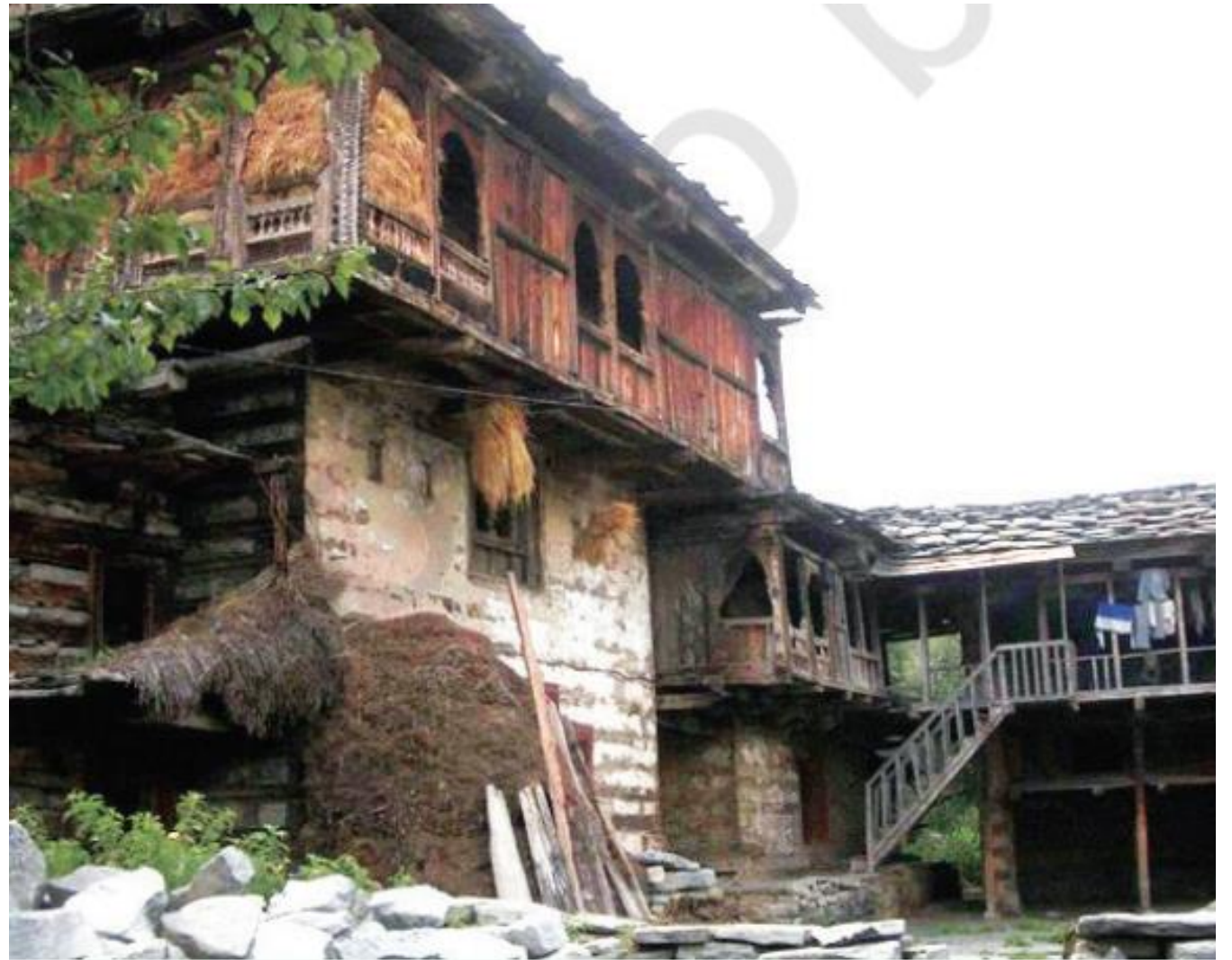
Fig. 1.6. Kath-kuni House, Himachal Pradesh
